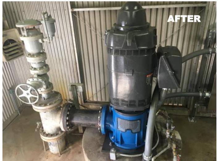
Teaming with Apollo, PumpTech's expert field installation crew and design engineers lead the effort to remove the existing 250Hp motor, angle drive and connections, discharge head, column, shafting, complete bowl assembly and cat walk next to the motor.
