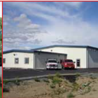
Moses Lake Eastern Branch Office
